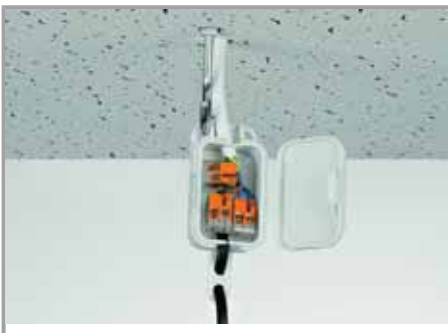
Pendant light connection in suspended ceilings
