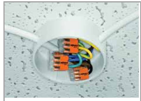
Lighting distribution in ceiling canopy
